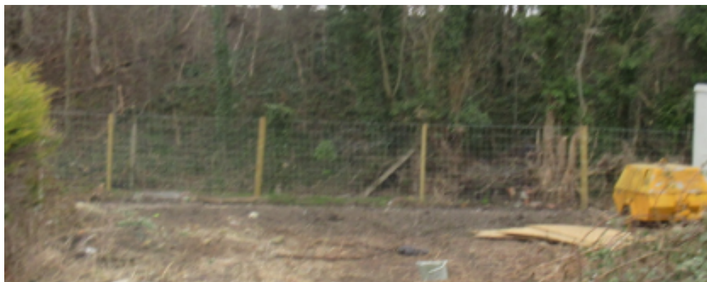
Post and wire fencing on the eastern boundary
