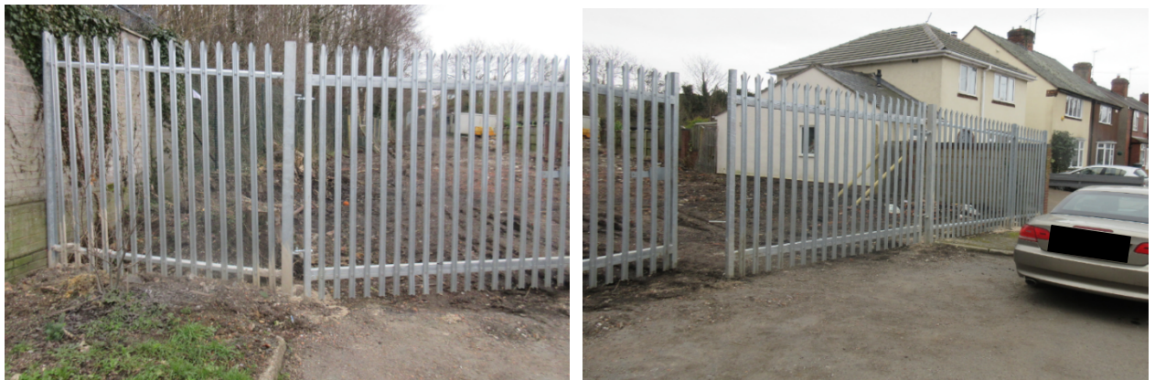
Photographs of fencing and gates on the frontage with Walgrove Road
